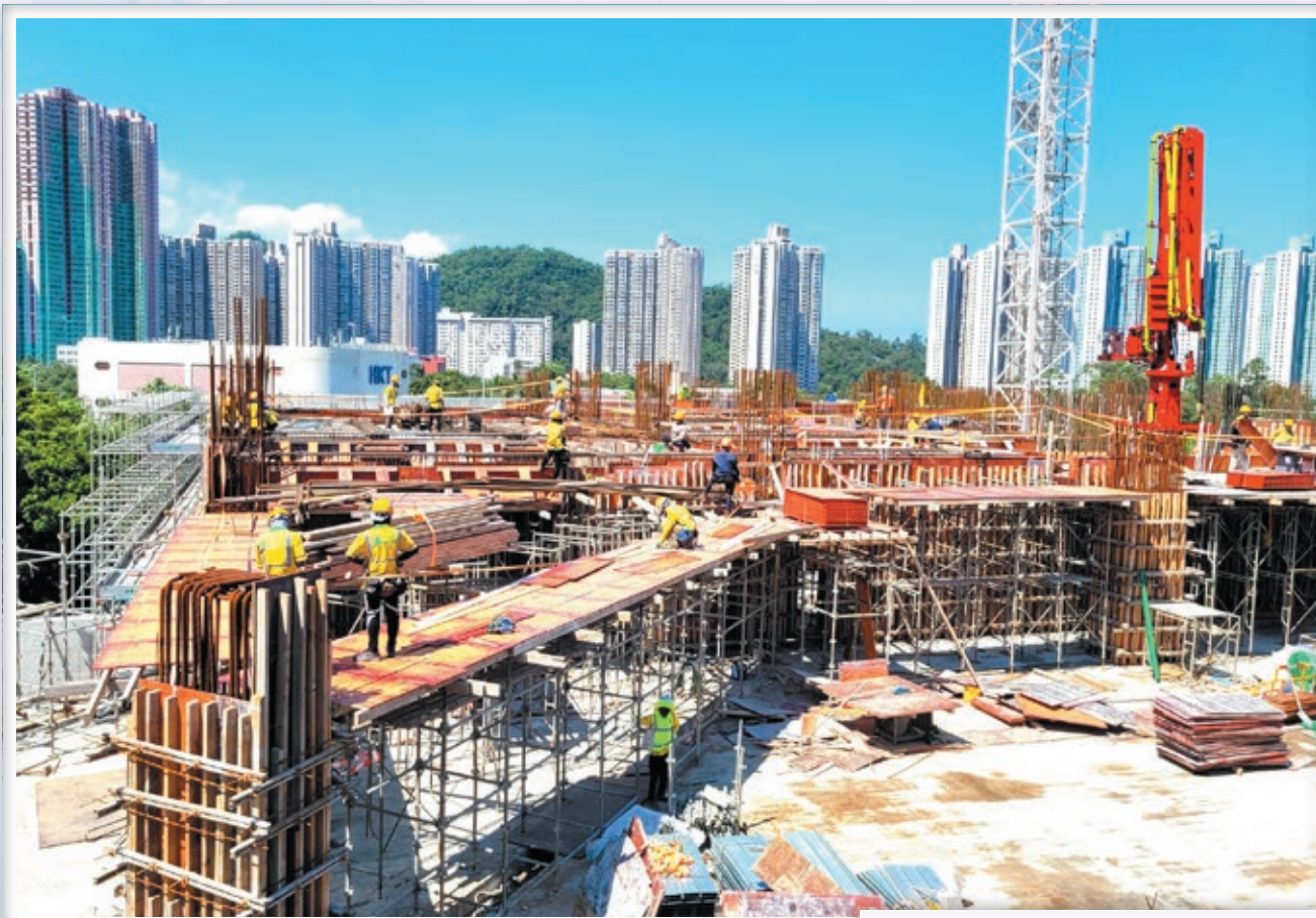
4 樓主入口樓面及相連架空道路 Fourth-floor main entrance floor and the connecting elevated roadway
